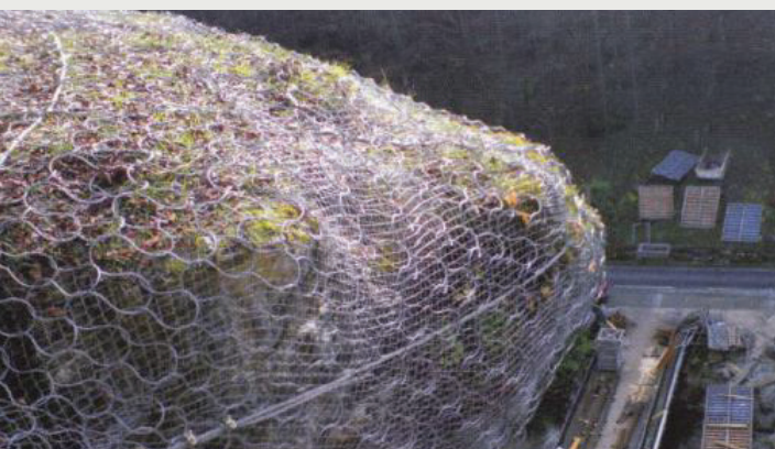
Heavy rock stabilization using Omega-Net.
