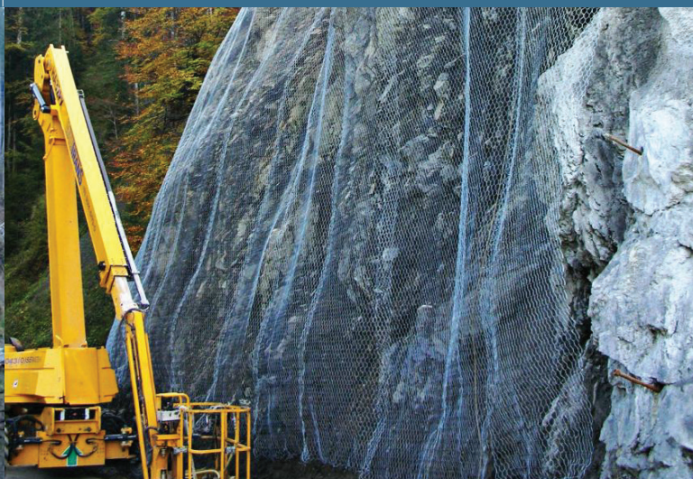
Example of a drape mesh system using hexagonal mesh.
