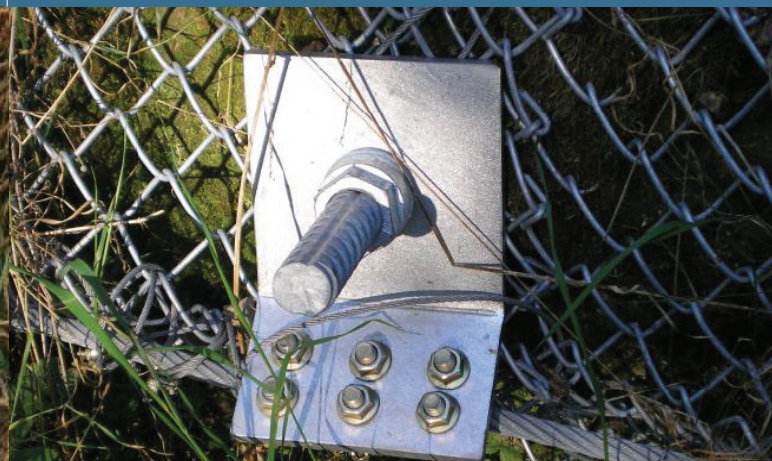
A non-positive/fixed connection to a boundary rope of a system.
