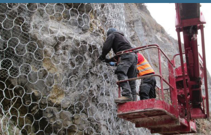
Installation of Omega-Net for slope stabilization.
