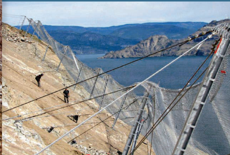
A lower energy attenuator system composed of High Performance Netting in combination with standard hinged posts and base plates.
