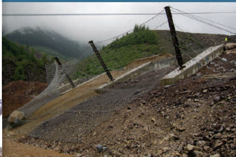
During the impact, the majority of the energy is absorbed during the initial contact with the upper section of the structure, but the projectile is allowed to progress through the system to the bottom portion of the net.
