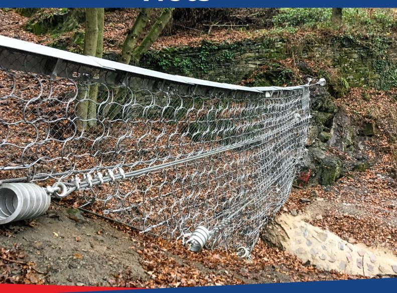
Gully nets are the simplest style of debris flow barrier. They are designed to be installed in topographically confined channels, typically up to approximately 15 m in width. The shape and gradient of the channel have a large influence on the retention capacity of the system. When in steep terrain, they are often used in cascading series to help successively remove the debris along the transportation zone of the debris flow.
