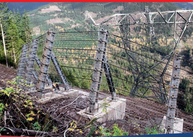
The lambda-frame Debris Catcher is a post-supported flexible-net barrier that can be installed in wide channels or along open slopes. Functionally, it is similar to the deltaframe system but can be used for larger events. The retention capacity of the system is controlled by the gradient of the slope and the height of the posts. An endlessly long system can be designed whereby independent sections are defined by internal anchoring of bearing ropes.
