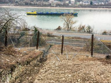
The shallow landslide barriers and modified rockfall catchment fences have the following advantages after professional planning and installation:
