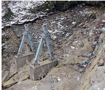
Debris flow barriers are designed on a site-to-site basis to protect infrastructure, utilities, buildings, and lives from debris flows and debris floods. Typical barriers are installed in run-out or deposition zones, close to the elements at risk that they protect or in series in the torrent channel. Each debris flow protection system is designed on a site-to-site basis, based on a thorough understanding of the debris flow characteristics.
