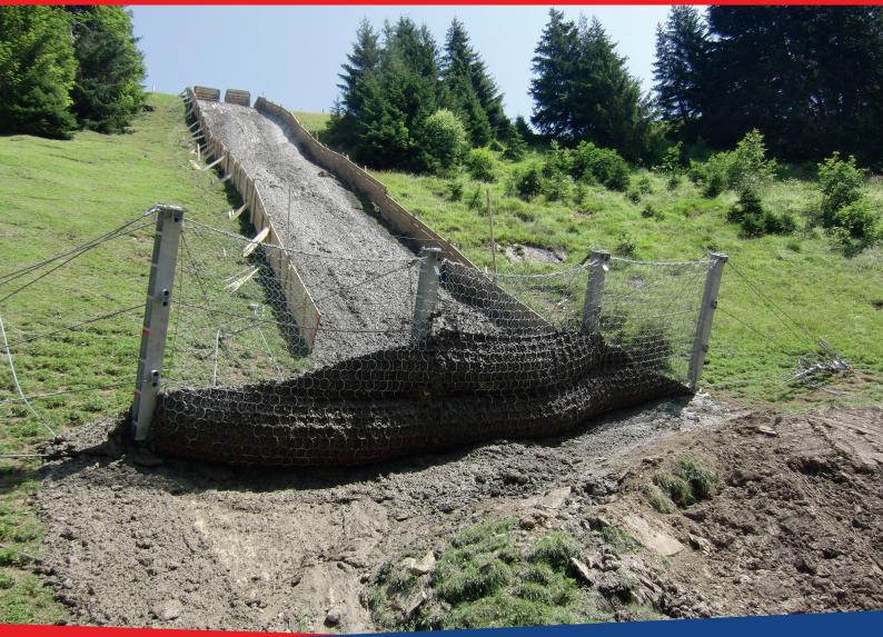
Shallow landslide barriers are systems evolved from rockfall catchment fences. As they are a post-supported system, they can be used in wide channels or along open slopes. These systems are especially suitable for the installation sites having difficult terrain.
